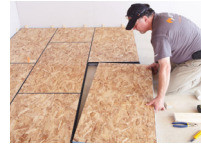
Install Subfloor with Brick Pattern
