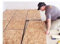
Install Subfloor with Brick Pattern
